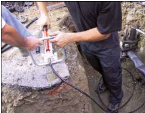
Pumping operation for pipe compressing
